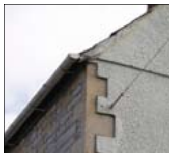
Render incorrectly pronounced beyond stone quoins
