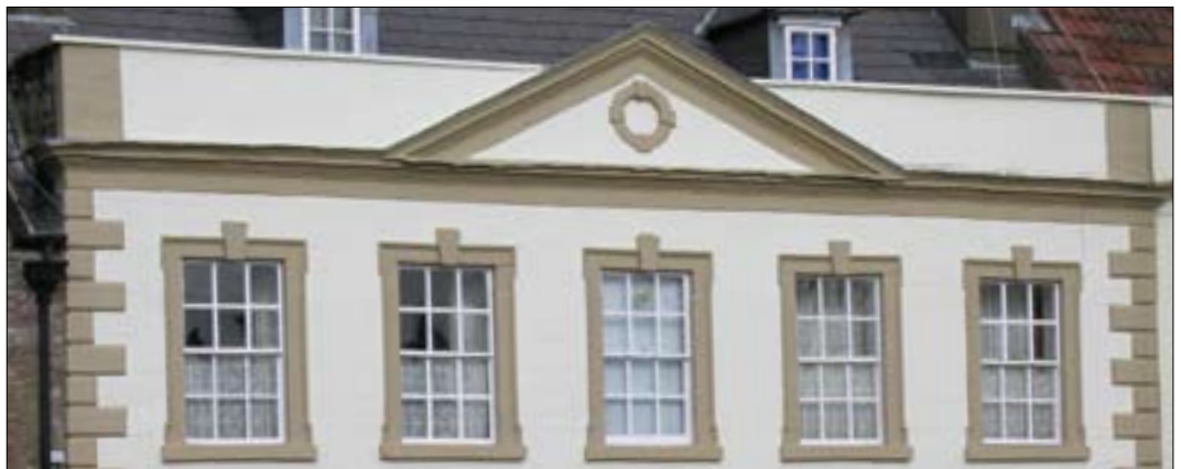
Stone quoins correctly pronounced from render
